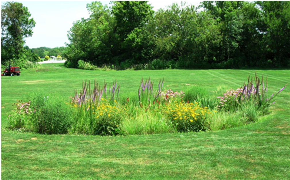
Picture 3 Green infrastructure, rain gardens taken from Susdrain
